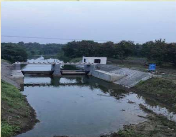
Ajraphata project with Rubber Dam (Water filled)
