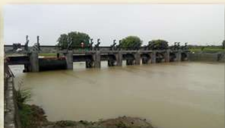
Deoli project: Automatic Gates in open and closed Position
