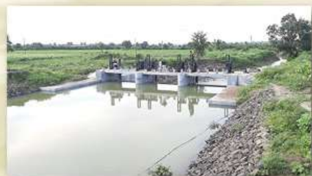
Sarwadi project: Automatic Gates in closed position,
